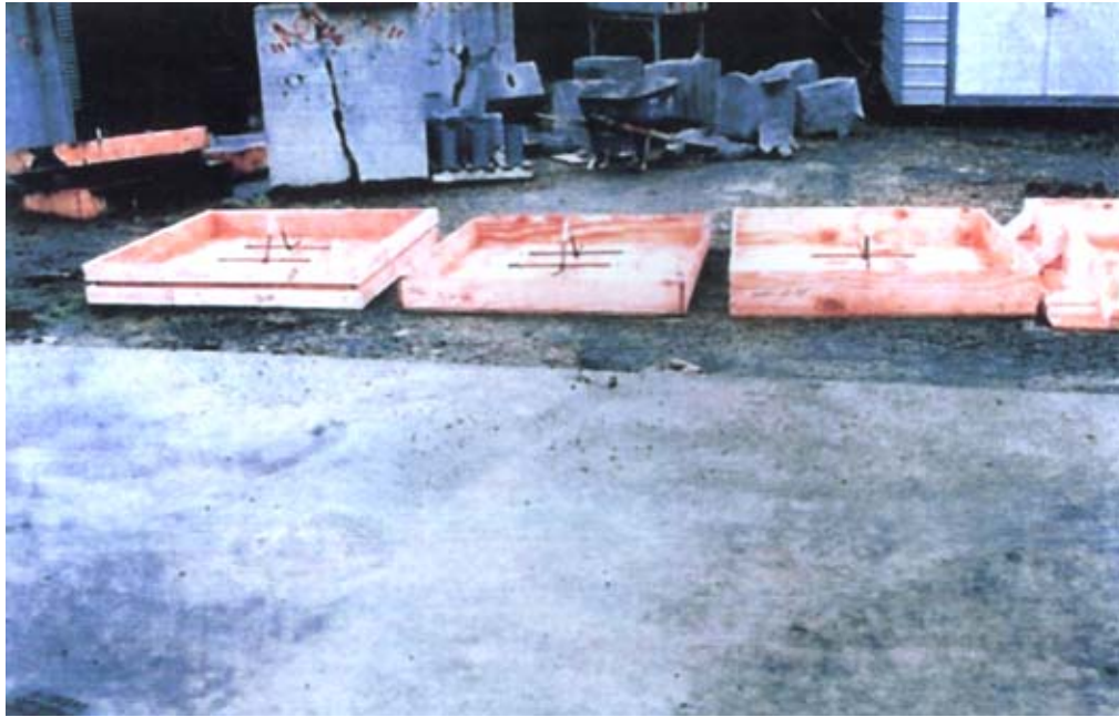
Photo 1. Forms before concrete placement
